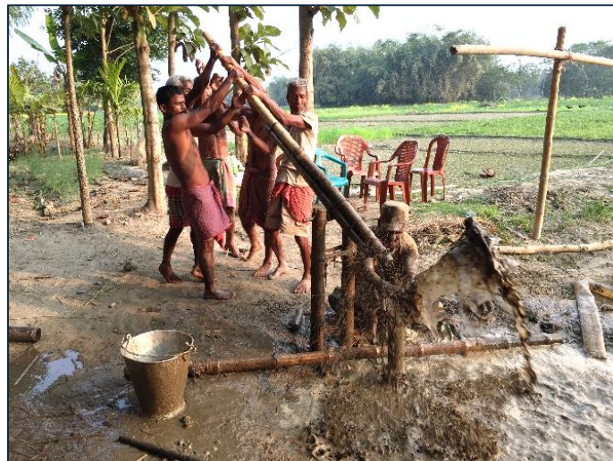
Installing shallow tubewell in Dholaguri, West Bengal
